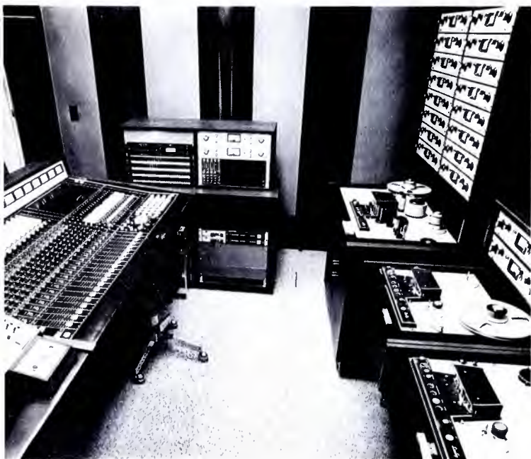
Custom console has 20 inputs and up to 16 outputs. It is capable of doing quadrasonic recordings. Note 16-track recorder. Studio was designed by Welton Jetton.
